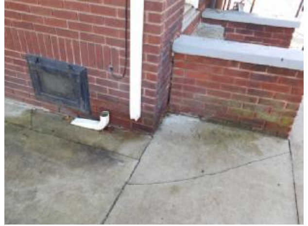
Improper Drainage
