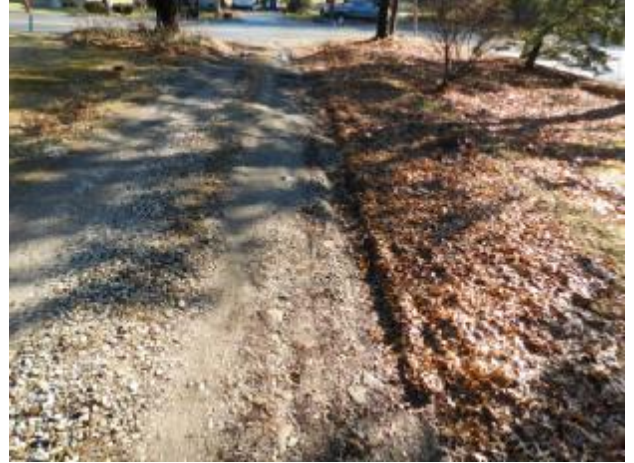
Ruts in driveway
