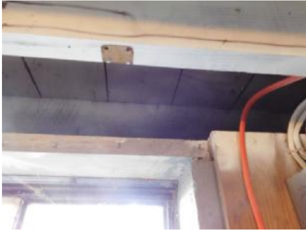
Missing insulation
