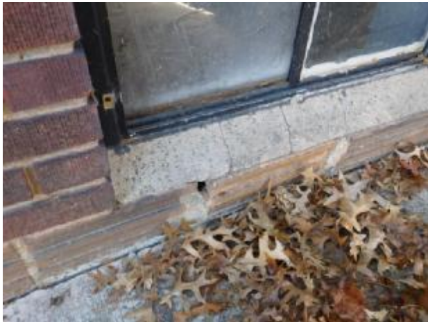
Missing mortar
